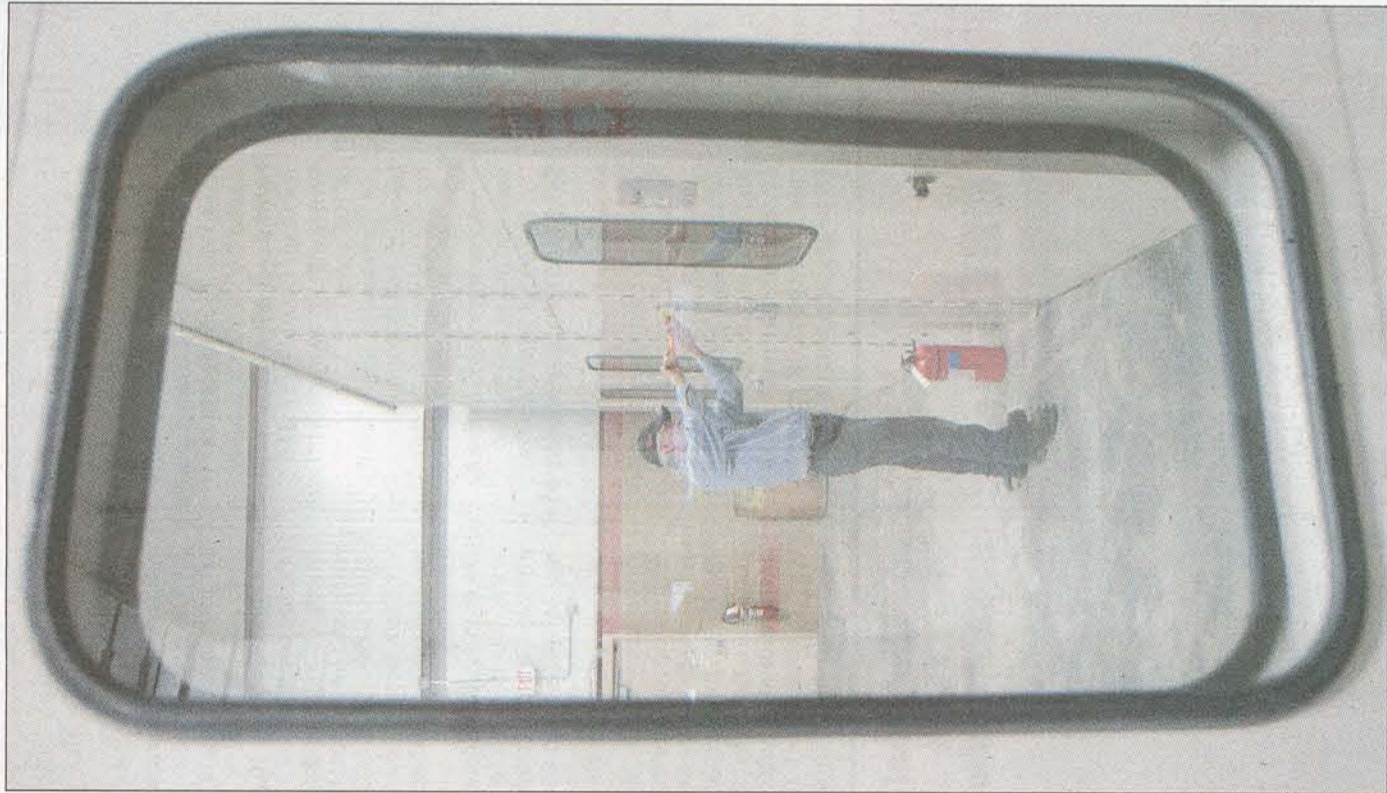
Above, Jeffrey Roda installs emergency stop switches in clean room cells used for engine and generator maintenance.
