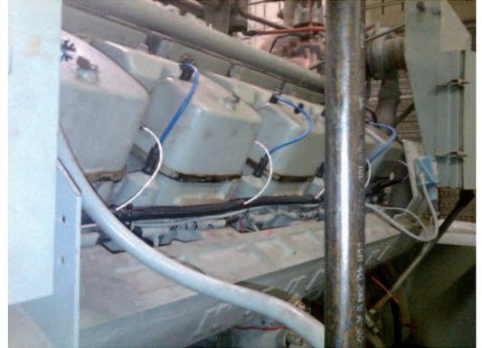
**Figure 3: Upgraded Waukesha L7042 GSI gas engine**
