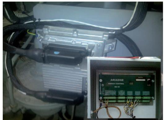
**Figure 4: HEINZMANN ARIADNE Knock control and PHLOX Ignition Control installed on Waukesha gas engine**
